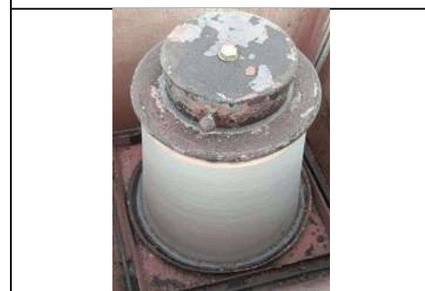
Fig. 11 Support Insulator.
