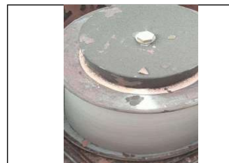
Fig. 12 Support Insulator.
